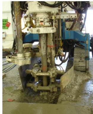
JET GROUTING DETAIL
