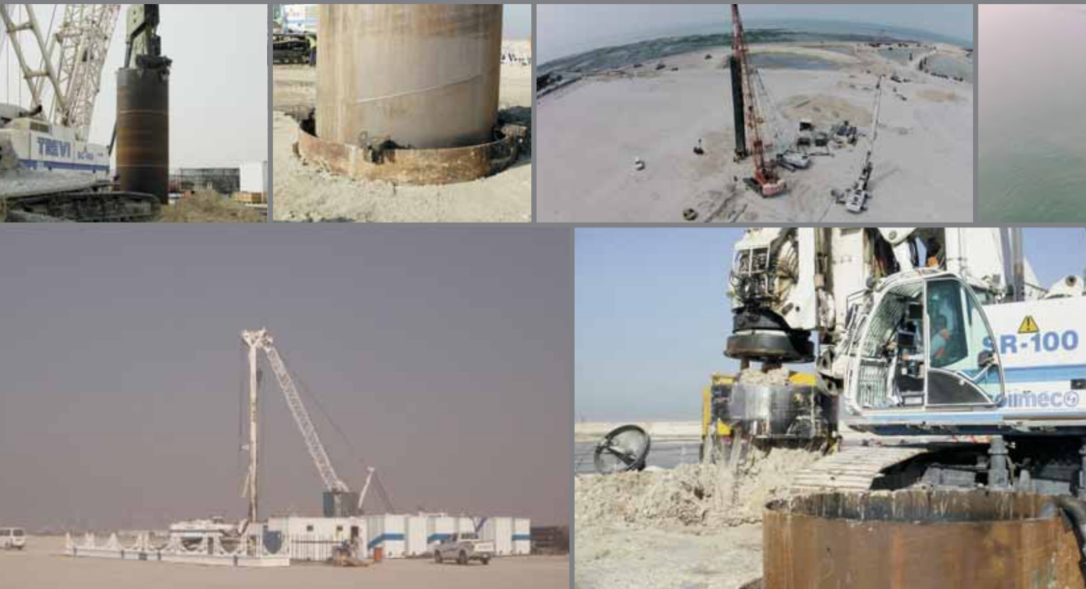
Area cantiere a terra / Onshore jobsite
