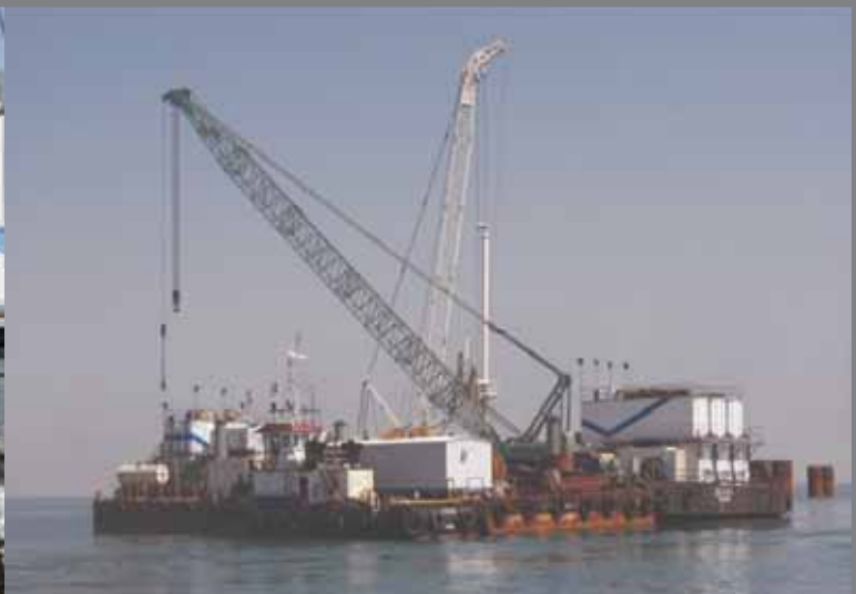
Area cantiere in mare / Offshore jobsite
