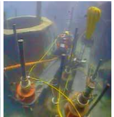
Tesatura e collaudo Testing and tensioning
