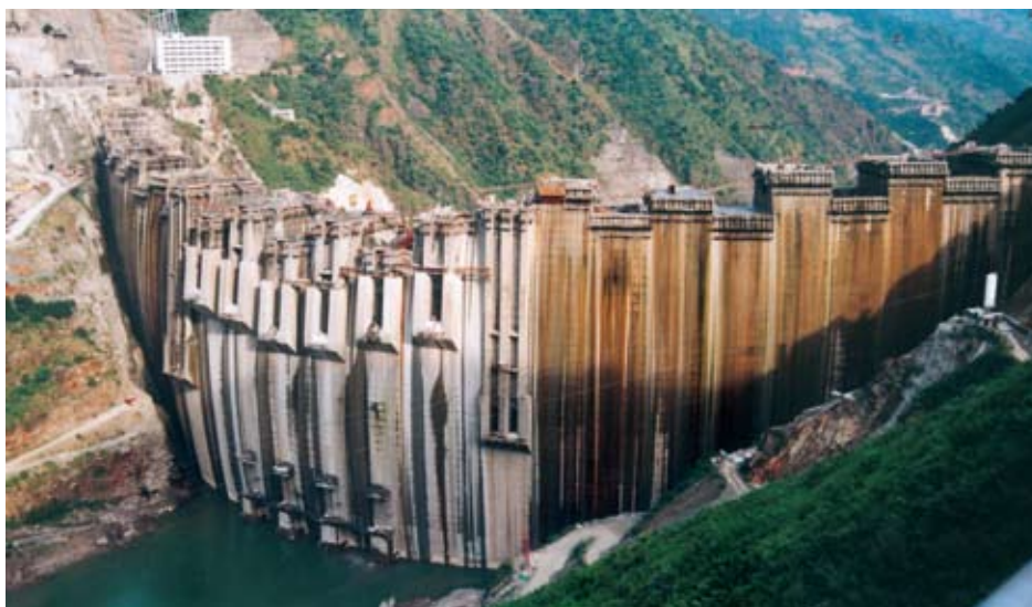
Ertan Dam (China).
