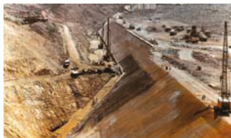
Khao Laem Dam (Thailand).
