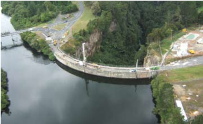
Arapuni Dam (New Zealand).
