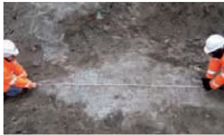
Colonne ellittiche di jet grouting. Elliptical jet grouting columns.
