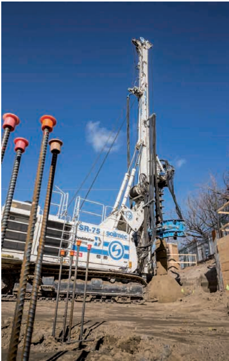
Soilmec SR-75 in configurazione CFA./Soilmec SR-75 in CFA configuration.
